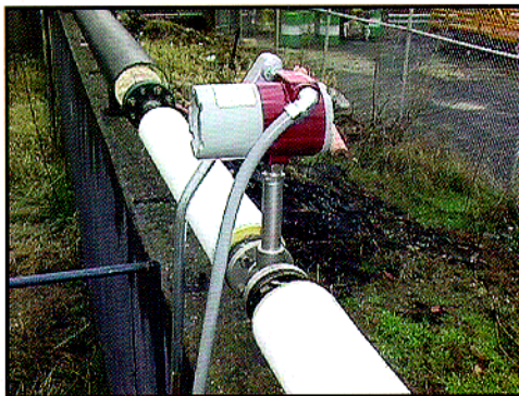
BOTH END USERS AND SYSTEM INTEGRATORS SAY INSTALLATIONS OF SIERRA INSTRUMENTS' MODEL 220/INNOVA MULTIVARIABLE VORTEX MASS FLOWMETERS ARE EASY AND ECONOMICAL.
