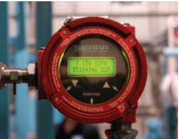
Sierra Steel-Mass™ 640S on a digester tank
