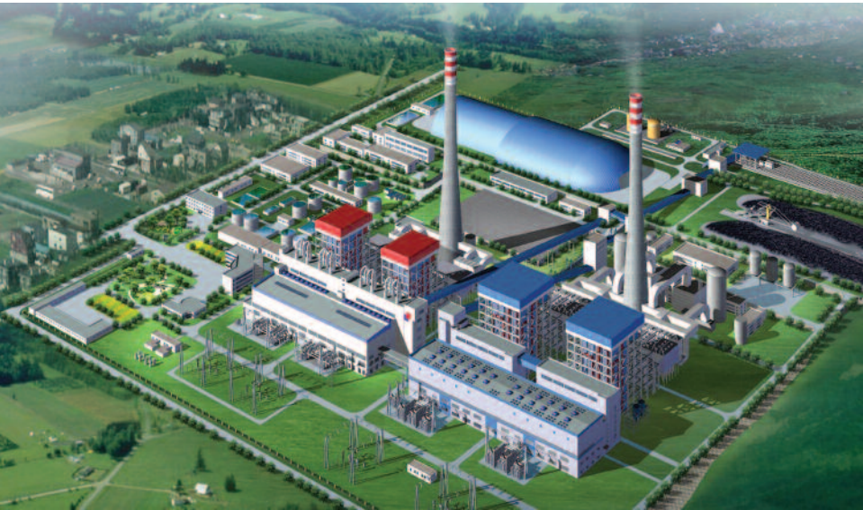
Yiyang coal-fired power plant in Yiyang, China
