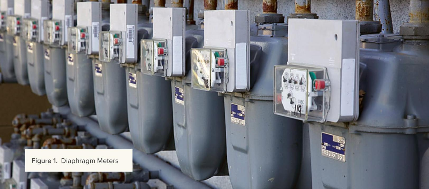
Figure 1. Diaphragm Meters
